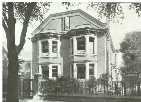
Garfield House (Senior School) was built in 1881 as a villa residence for Mr James Carver. In 1901, it became a Convent for the Sisters of the Sacred Heart. Tales of ghostly nuns have been told ever since!
